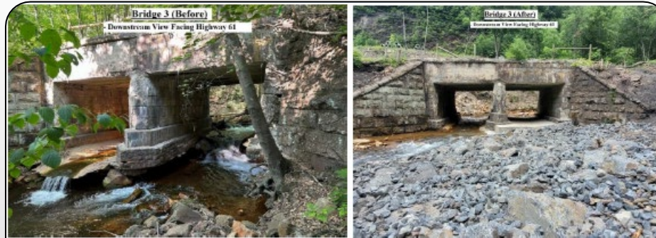
BEFORE/AFTER OF RAILROAD BRIDGE REHABILITATION
