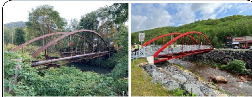
BEFORE/AFTER OF REHABILITATED AND RELOCATED 1878 HISTORIC BOWSTRING TRUSS
