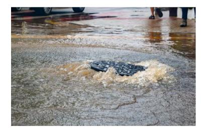
Inflow and Infiltration is water that enters the sanitary sewer. During times of high rainfall, I & I rates increase and can cause wastewater treatment problems as well as flooding in the sanitary sewer system. The Township actively pursues and addresses I & I to reduce the daily flow to the treatment plant.
